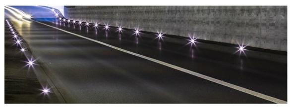
Figure 5: LED Floor Guidance Lights
