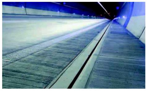
Figure 13 Slotted Channel for Drainage
